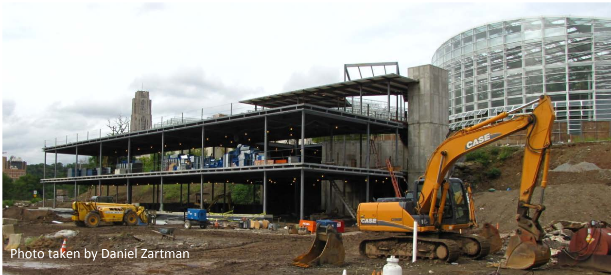
Figure 3 - Concrete and steel superstructure taken September 7, 2011.
